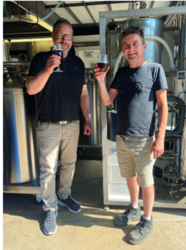
Kim Dalum (L) and Eddie Gadd toast the successful installation of the equipment at Gadd's Ramsgate Brewery, August 2022
